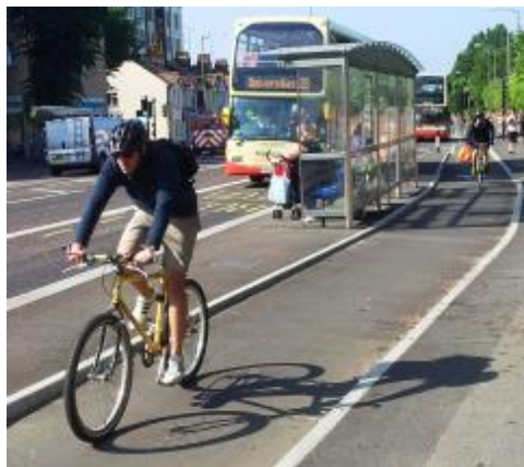
Figure 4.1 A floating island bus stop on Lewes Road, Brighton reduces the potential for conflict between cyclists and bus es.
