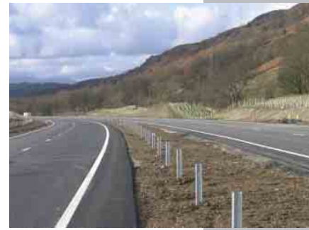
New dual carriageway section of A590 past Ayside, Cumbria, prior to opening
