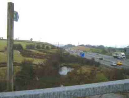
M65 north of Tockholes, Lancashire, showing footpath diversion alongside motorway to cross at minor road bridge from which the picture is taken.
